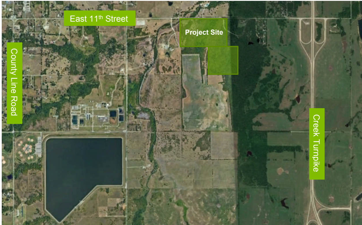
Figure 1. 2022 Aerial Photograph/Project Site Outline.
