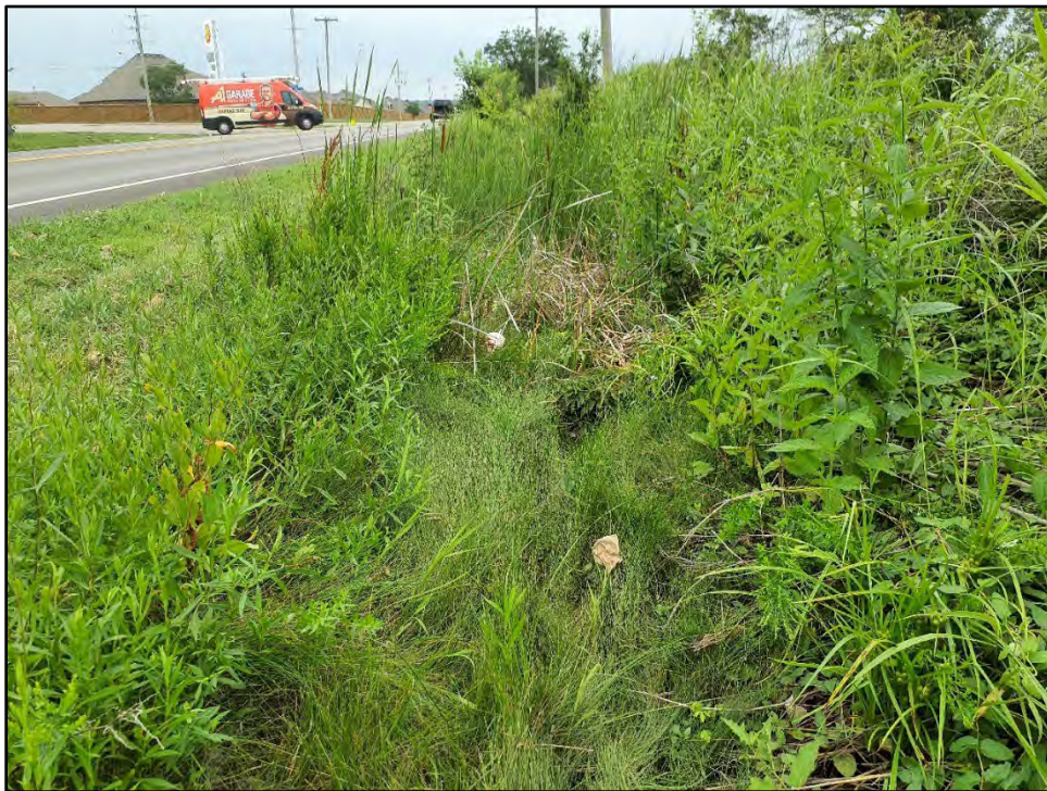
Figure A20. Representative photo of ephemeral stream SA015 (roadside ditch) within the project area, facing upstream.
