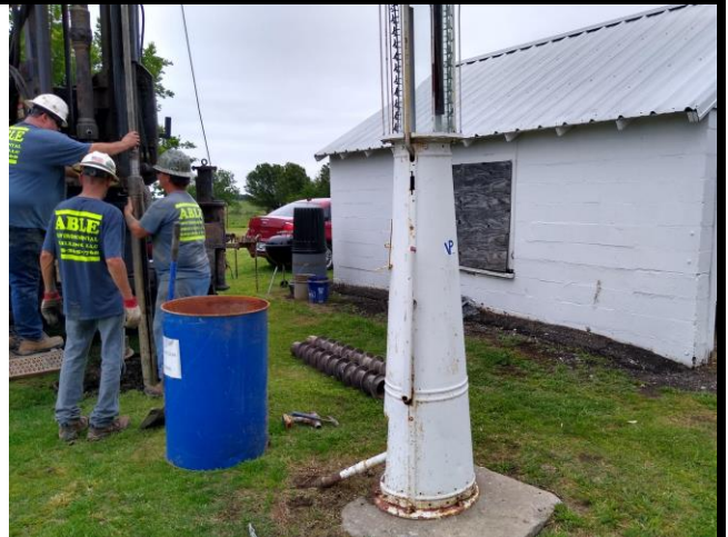
Typical drilling activities and the fuel dispenser.
