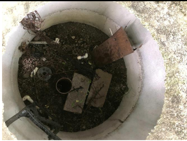
The inside of the suspect groundwater well.
