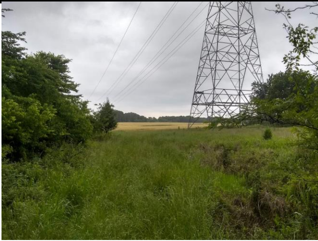
A typical view of Section 3 from the west, looking east.
