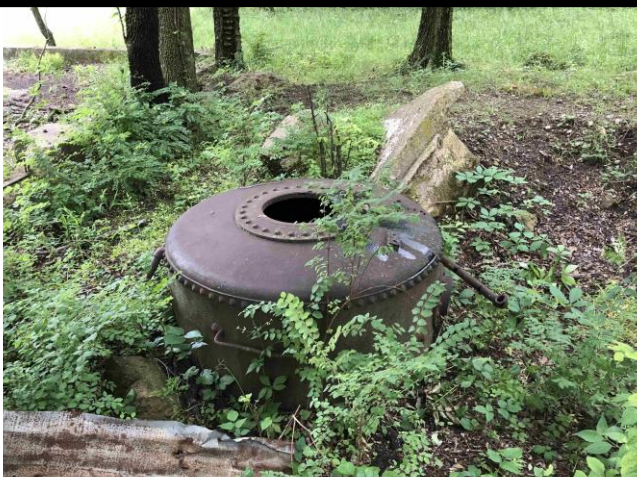
An underground storage tank located south of the scale house.
