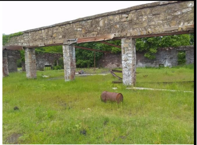
The coal storage building from the east, looking southwest.
