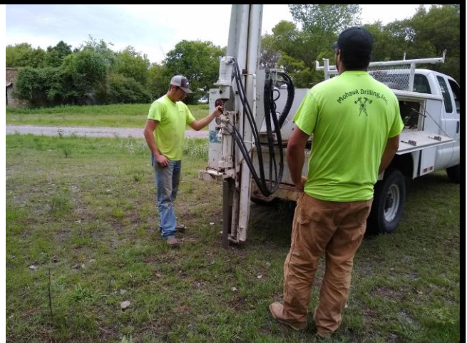
Typical subsoil sampling activities.
